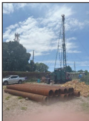
JACISERA Park Irrigation project
